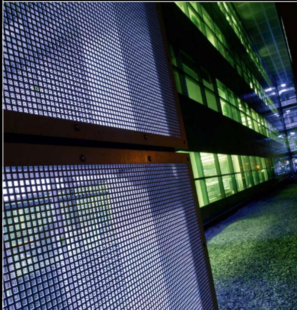
More than 1.3 square kilometres of precision perforated aluminium from RMIG Group is being used to provide a distinctive and decorative exterior cladding solution at White Star House.
